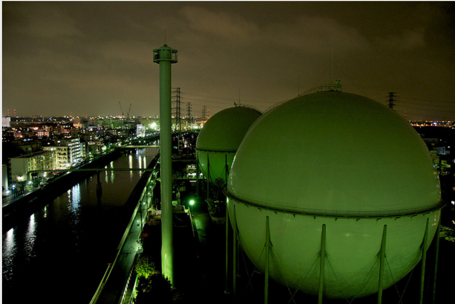
Shinichi Higashi, Gas Tank. CC BY NC SA
